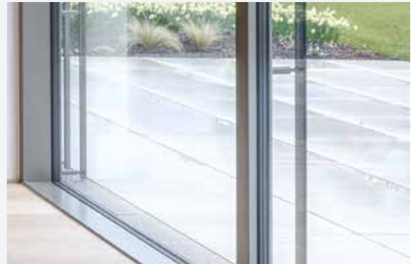
Fixed glazing in the threshold
