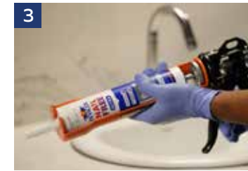
3 Load cartridge into the gun
