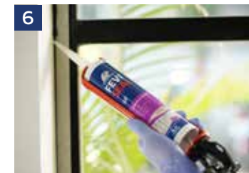
6 Fill the sealant into the gap
