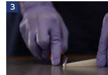
3 Cut the nozzle in 45 degree equal to the gap width
