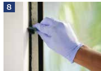
8 Remove masking tape before drying
