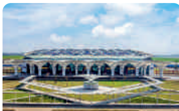
International Airport - Jabalpur
