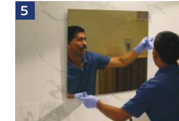
Bond substrates & provide support
