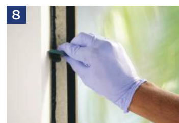
8 Remove masking tape before drying
