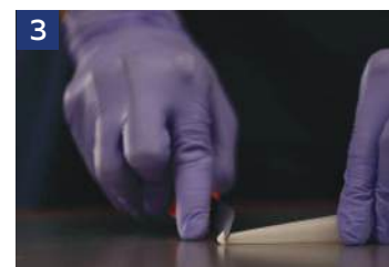
3 Cut the nozzle in 45 degree equal to the gap width
