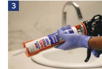
Load cartridge into the gun
