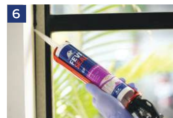
6 Fill the sealant into the gap
