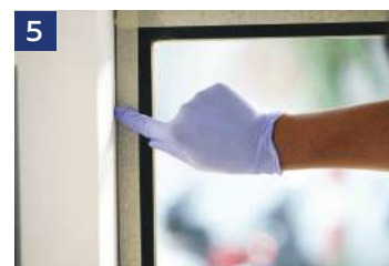
5 Fix the masking tape on both sides
