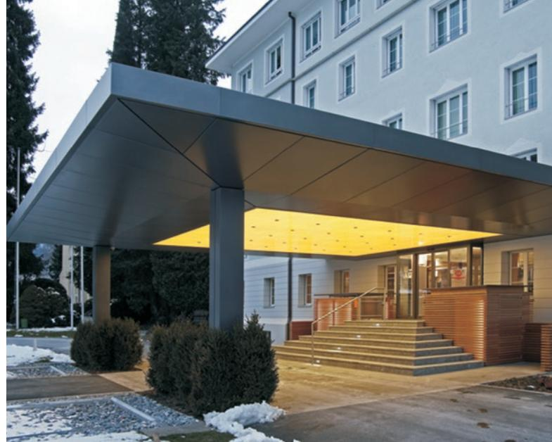
The steel construction of the above canopy roof has been cladded with aluminium sheets.
